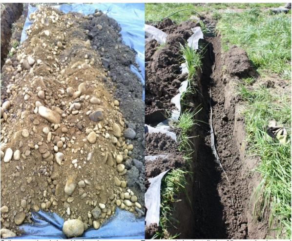
Soil removed and placed in three layers.
